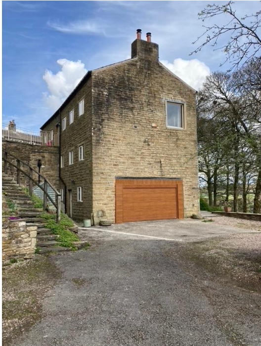
Photo 2: showing the site levels
